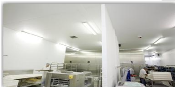
Proper lighting facility in the work area
